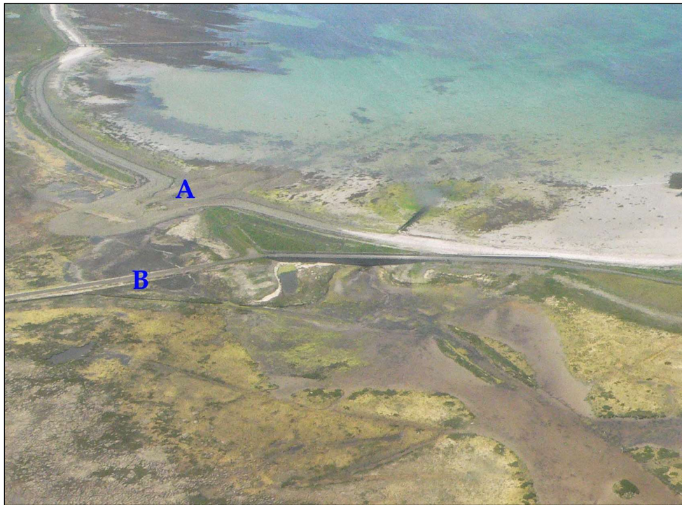
Figure 4.1: Aerial image of breaching, overwash (A) resulting in flooding of road (B) enhanced by low-lying and landward sloping interior (negative gradient). SW of Cleat, Little Sea, Sanday, Orkney.
